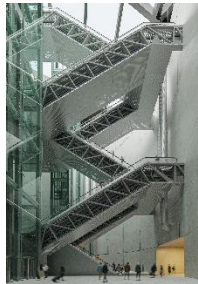
SANTO OVIDIO NORTH STATION, VILA NOVA DE GAIA
